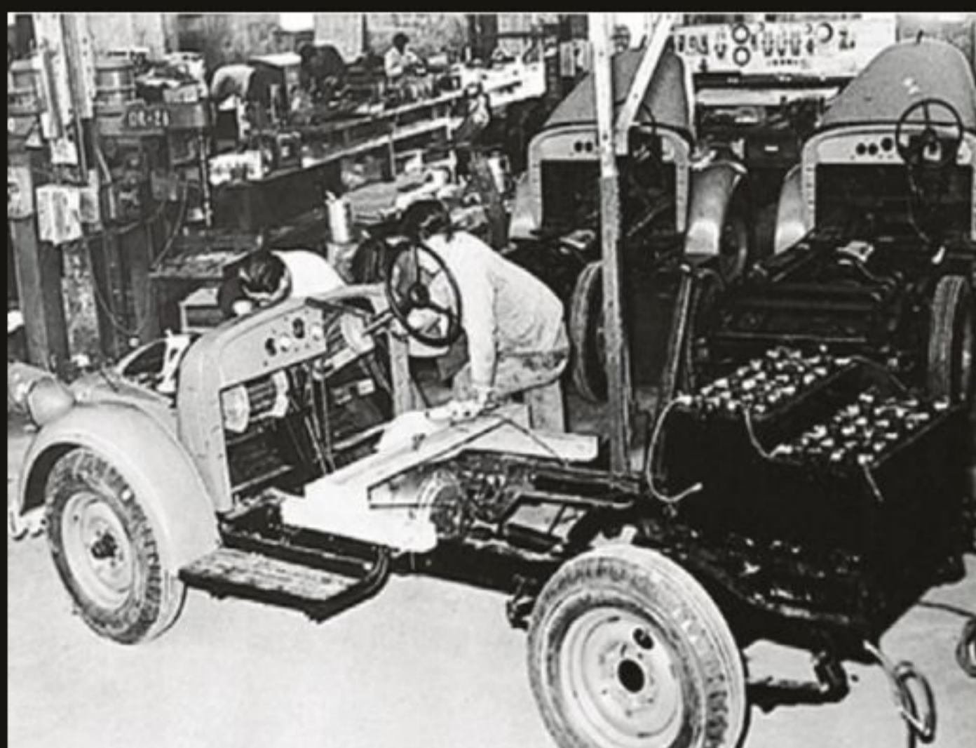
The Denso No 1 was a modified Toyopet SD, which was equipped with an electric powertrain.
